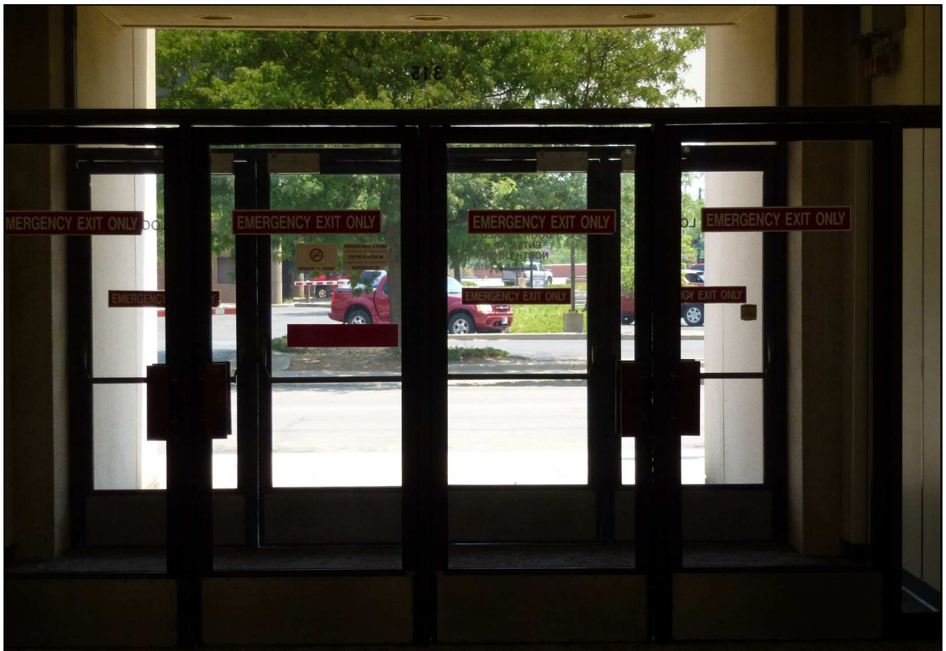
05. Elkhart Courts Bldg Emergency Exit
