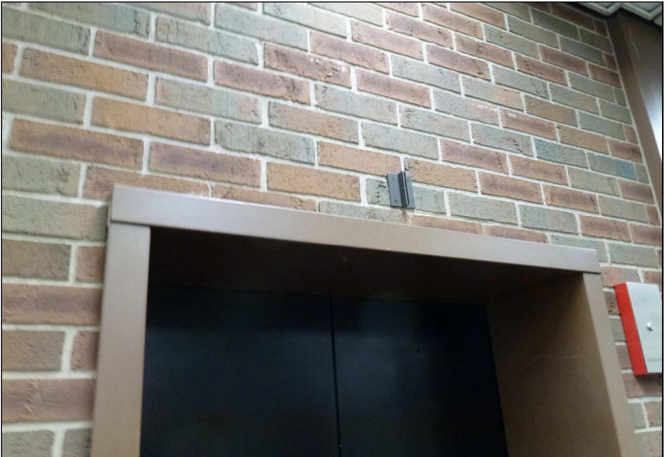
10. Elkhart Courts Bldg Elevator Signage
