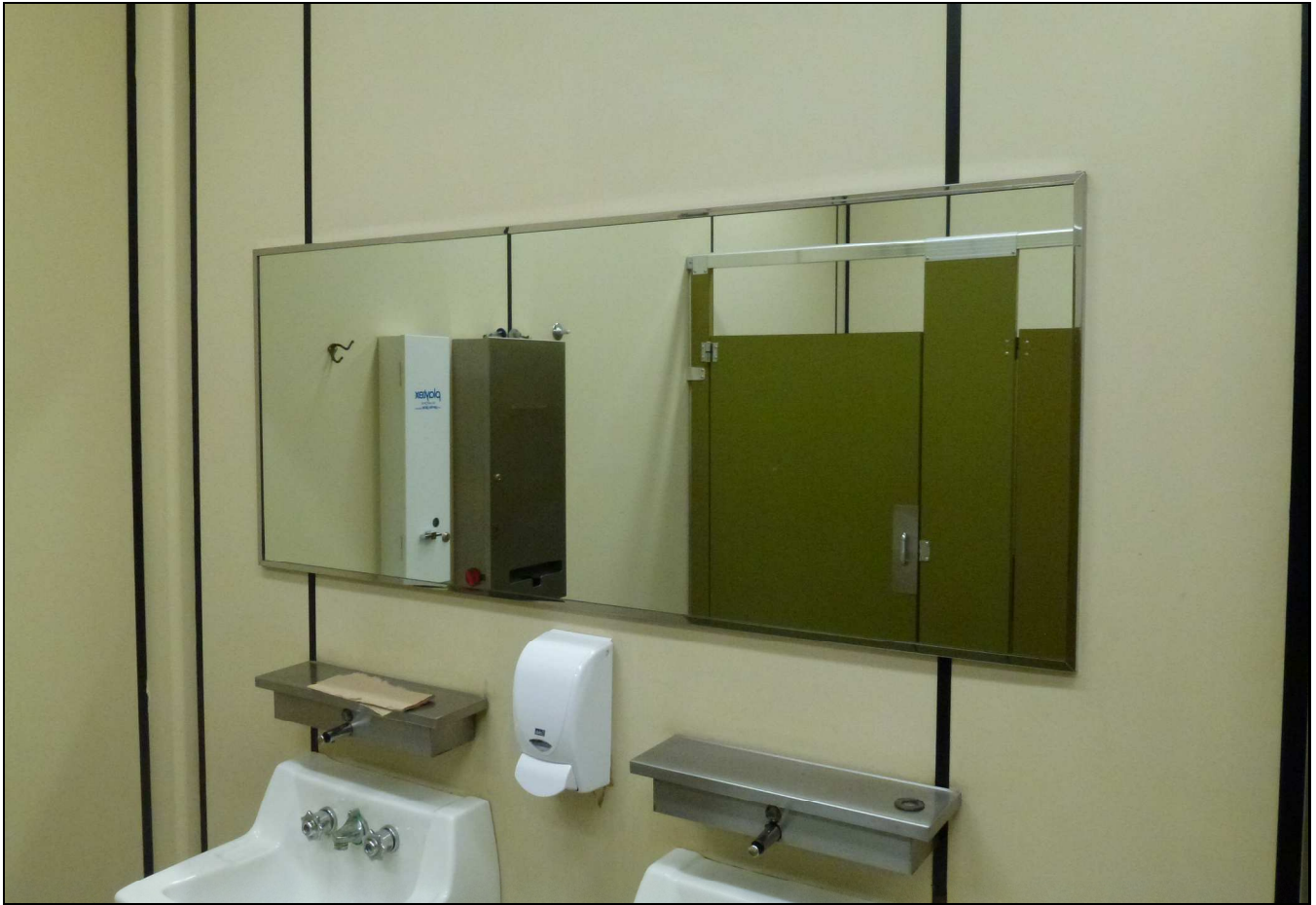
15. Elkhart Courts Bldg Bathroom Mirror
